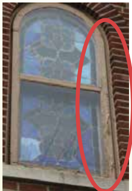
DETERIORATED WOOD/PAINT
