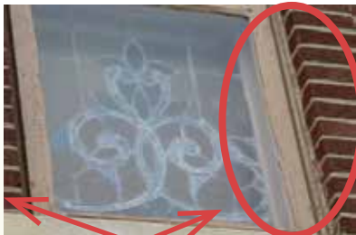
DETERIORATED WOOD/PAINT
